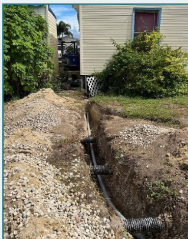
Upper right: Aaron demonstrates the new e-bike to William McNeil. Bottom right: The new electric service lateral to William's house.
